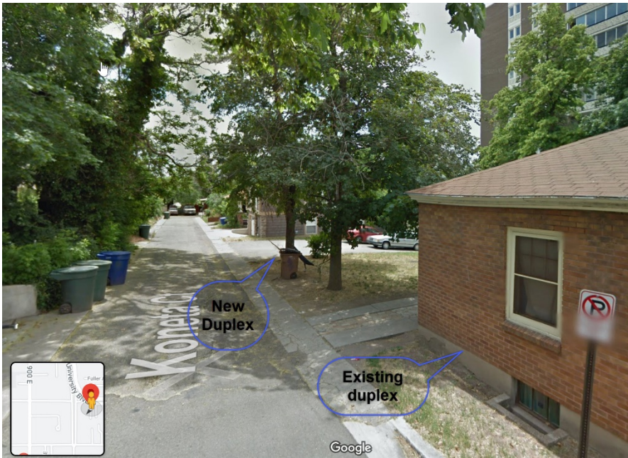
Looking south along Koneta Court, project site on right.
